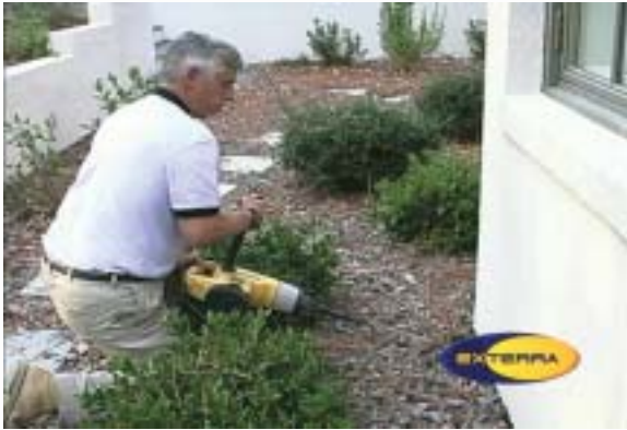
Barrier Application Preparation
